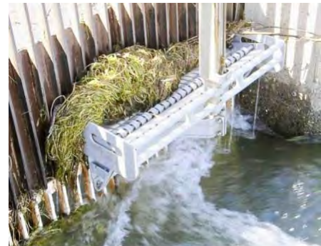
Automatic Trash Rake Facility in Balingasa Creek
