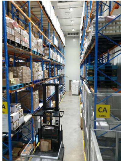
Cold Room, 2 to 8 deg C
