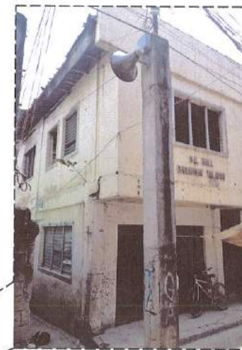
EXISTING STRUCTURE FOR DEMOLITION
