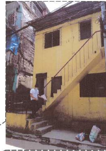
EXISTING STRUCTURE FOR DEMOLITION
