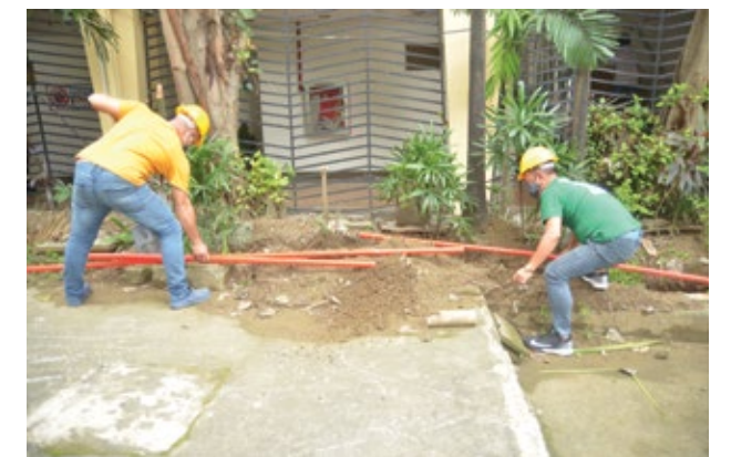
Network Cabling in Quezon City Hall
