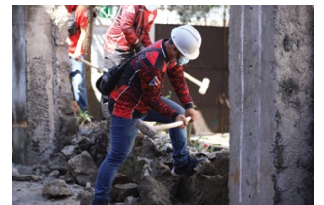
Clearing of road obstruction
