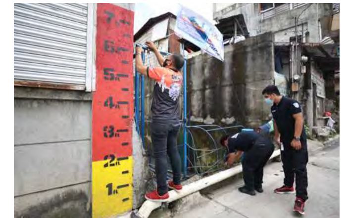
Installation of slope protection and flood control markers
