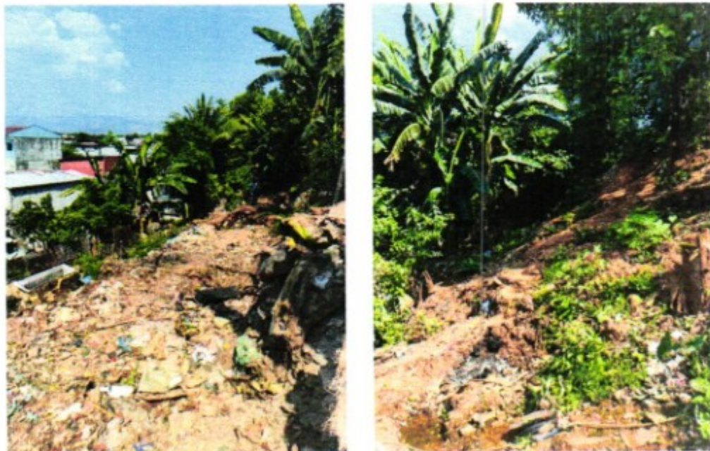
Figure 1 Existing Site Condition
